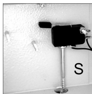
Figure 28 - Assembly of tamper for the MP500/16 control panel
